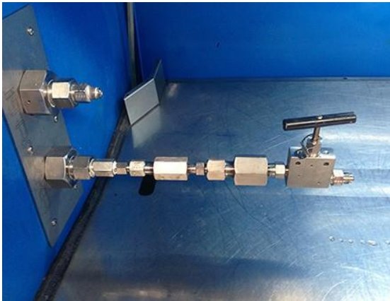
Figure 3: Set up for hydrostatic pressure test showing various pipe fittings/sizes
